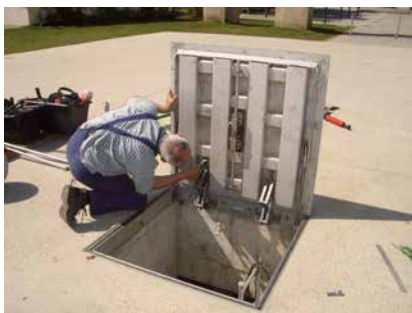
Retrofitted installation of an emergency escape
